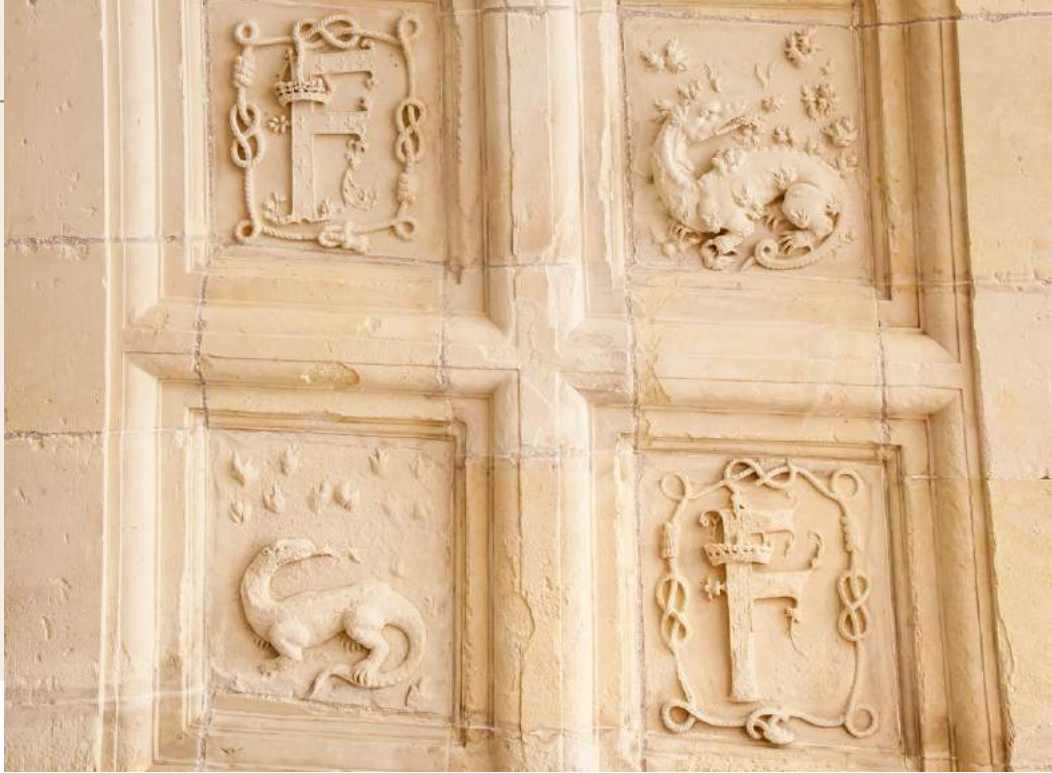
View of the sculpted vaults on the second floor
